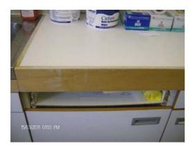
The wooden surround in the dirty utility is not acceptable and should be replaced as wood cannot be cleaned effectively and this can cause a potential risk of contamination.
