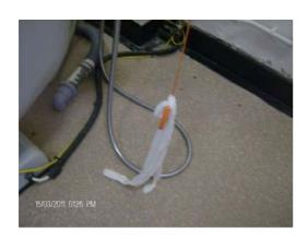
We found a number of bandages attached to the emergency call strings as they were not a suitable length; this is unacceptable due to the risk of contamination.
