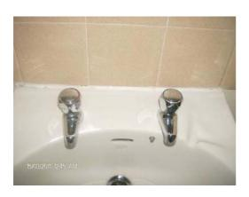
rooms are not clinical hand washing sinks and do not conform to Health Technical Memorandum (HTM) 64. All clinical hand washing sinks should have elbow, knee or sensor operated taps. In order to minimise the potential infection control risk taps should be easy to turn on and off without contaminating hands. The current taps should therefore be replaced.
